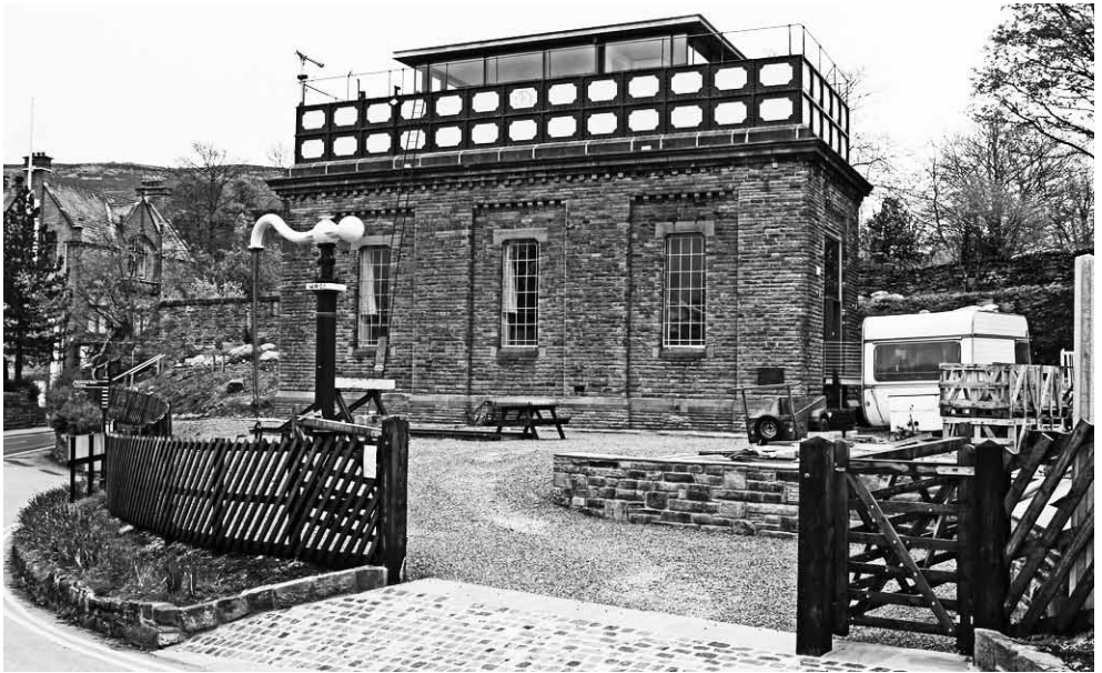
Above: Settle Station Water Tower is 10.26m high. The Eden Brows steel & concrete piles go down 20m. Photo: Mark Rand
